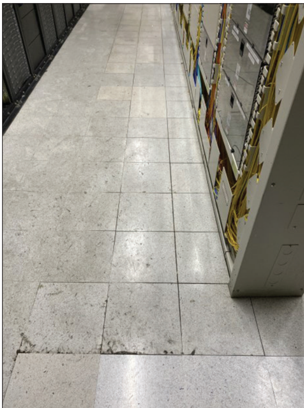
Figure 1: Deteriorating floor in cable company server room
