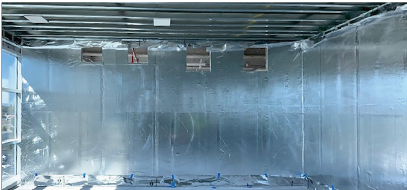
Figure 3: Example of ICS/ICD-705 RF shielding barrier installation
