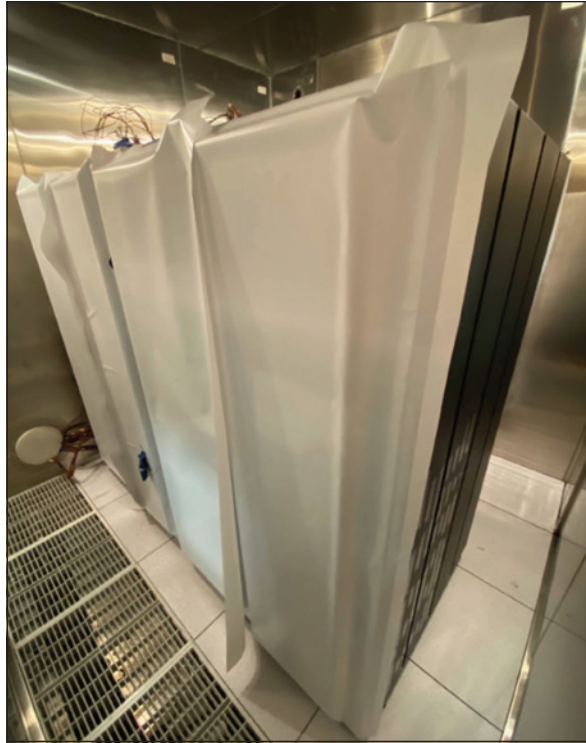
Figure 6: Blocked ventilation test
