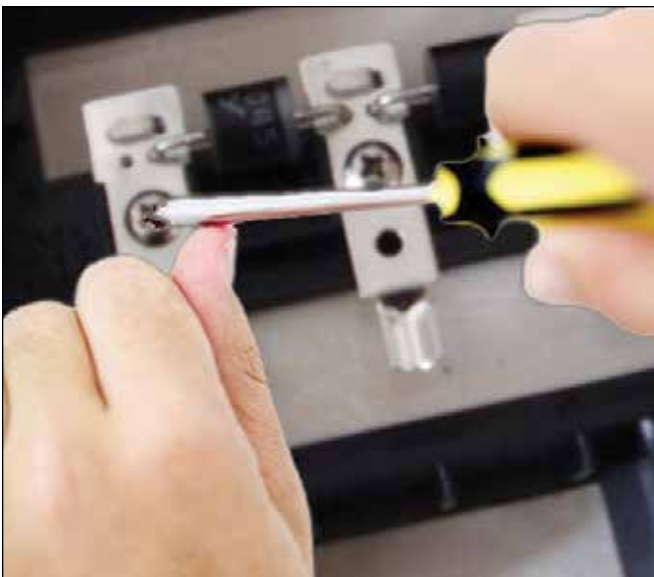
Figure 4: HMM event between a screwdriver and a screw that is part of an electrical installation in the junction box.
